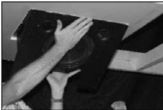
Figure 7: Installing the subwoofer using the ledge to temporarily secure it.
